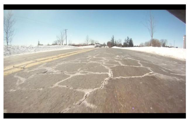
Figure 4: View, looking westbound, at the road surface of Sunningdale Road in London, Ontario, taken by the video camera located beneath the front bumper of the test vehicle.
