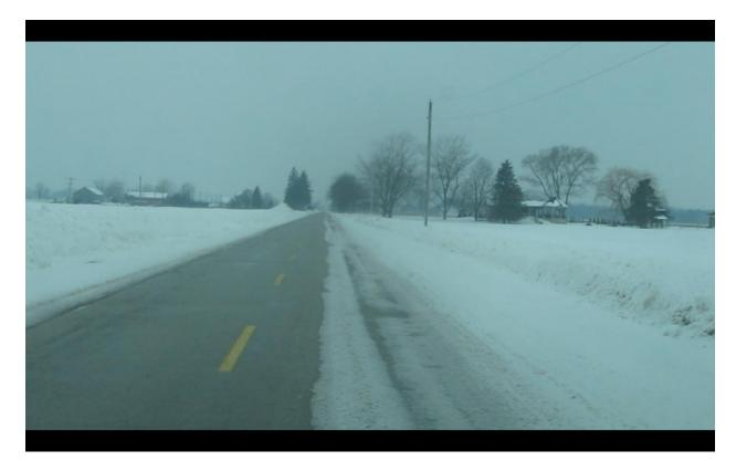
Figure 3: View, looking west, along Oil Springs Line showing the hardened snow and ice located on the right half of the westbound lane. This was the condition of the road at the time that the motion data was obtained with the test vehicle.
