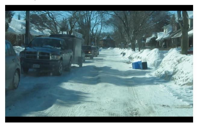
Figure 2: View, looking west, along McKenzie Avenue in Old-South, London, Ontario, showing the deep ruts caused by unplowed snow that had been compressed into solid ice and snow on the road surface. This was the condition of the road at the time that the data was captured.
