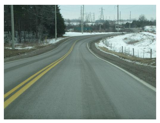
Figure 1: View, looking southbound at the S-Curve of Clarke Road north of Fanshawe Park Road in London, Ontario, showing the horizontal and vertical alignments of the road.
